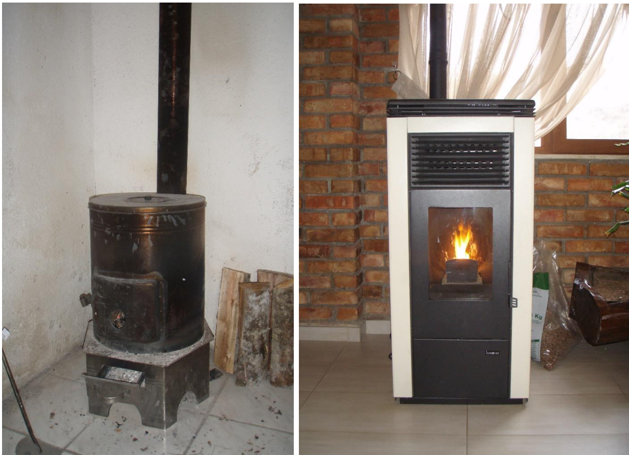
Old wood stove in an office (left) and pellet stove (right)
